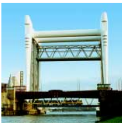
Positioning even in harsh environments: Bearing-less HÜBNER HG 18 Digital-Tachos measure and synchronize the speed of the drives on this vertical lift railway bridge near Rotterdam (➔ Figure 25 on page 19).
